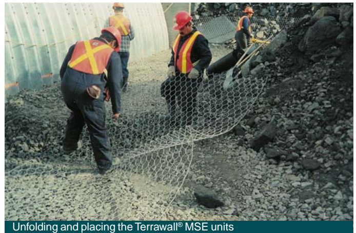
Unfolding and placing the Terrawall® MSE units
