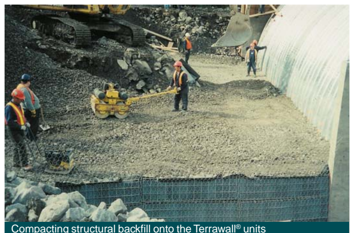
Compacting structural backfill onto the Terrawall® units
